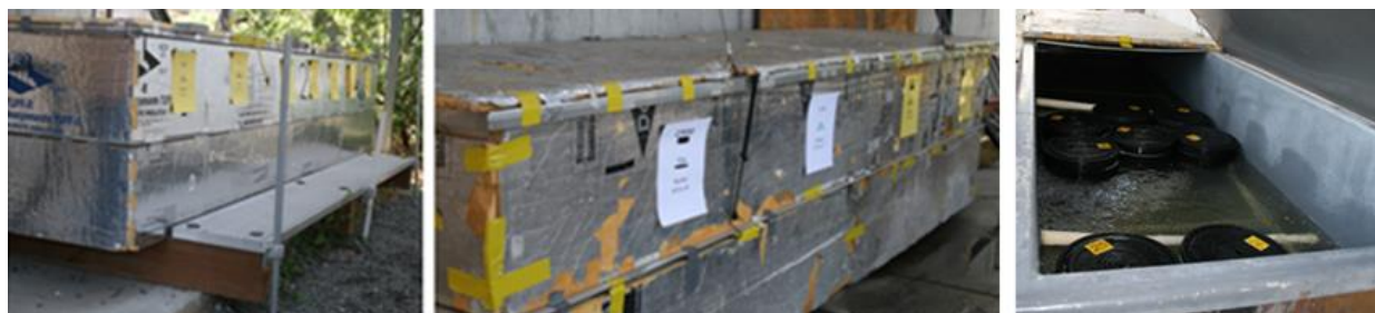
Figure16. Large Insulated Tanks for Holding Transport Buckets at the JDA SMF. Holding tanks are plumbed to allow flowing river water to pass through the tanks, each of which holds a maximum of 36 transport buckets.
