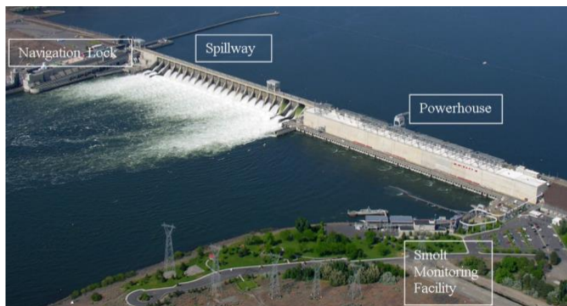
Figure 1. Aerial Photograph of McNary Dam. The Washington shore is on the upper left side of the picture (north) and the Oregon shore with the Smolt Monitoring Facility is on the lower right side (south).
