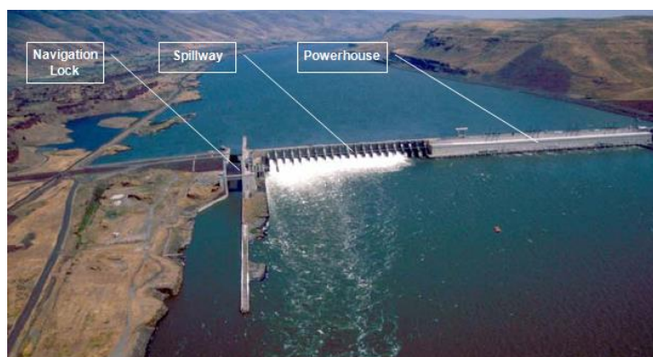
Figure 2. Aerial Photograph of John Day Dam from a Downstream Location. The Washington shore is on the left side of the picture (north) and the Oregon shore upstream of the Smolt Monitoring Facility is on the right side (south).
